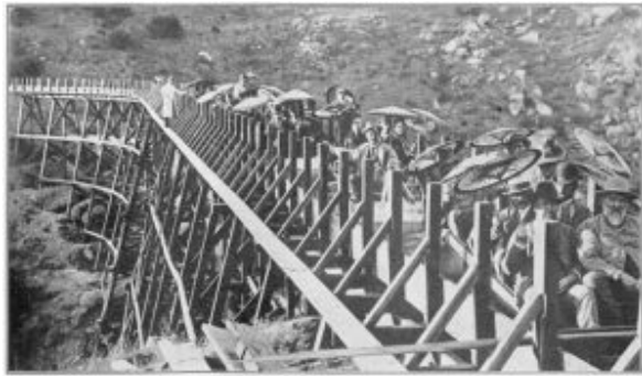
DEDICATION OF THE SAN DIEGO FLUME. The man at the extreme right is Governor Waterman. The man in the second row wearing a straw hat is W. E. Robinson, one of the originators of the enterprise.
