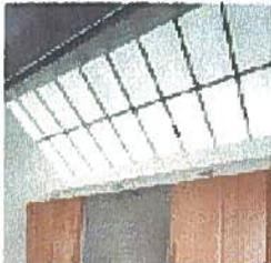
Translucent wall and Roof Assemblies shall be a double-faced, insulated, translucent fiberglass sandwich panel product based on the performance specifications of Kalwall.
