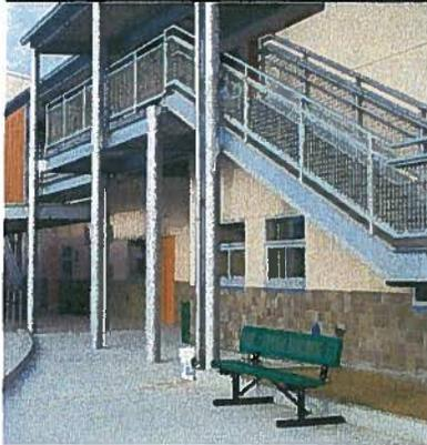
Exterior handrails and associated components to have galvanized finish per the American Galvanizing Institute's recommendations, and specifications to allow District ability to reject poorly finished, 'burred', etc applications. Metal shall be free from pitting, seam marks, roller marks, stains, discolorations, and other imperfections where exposed to view on finished units.
