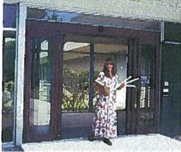
Automatic doors are to be by Stanley. Whenever possible, utilize telescoping doors for increased wear-ability and decreased door intrusion into the path of travel.
