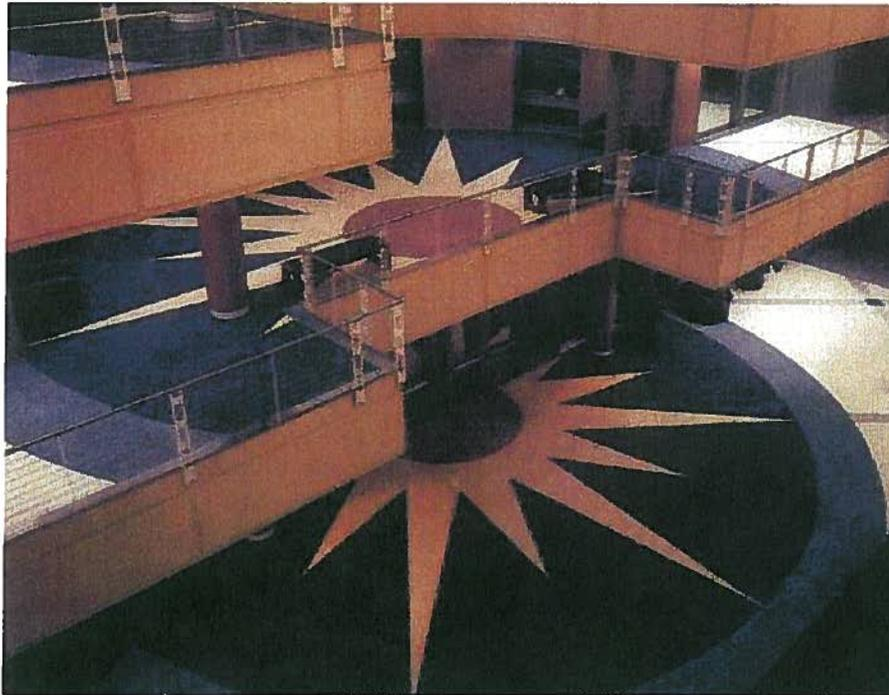
**Disadvantages**-System is dependent on a good slab floor. Colors are more restrictive and harder to control than with an epoxy matrix. *Cement matrix is not resistant to the acidity of urine or other chemicals in cleaning compounds and therefore will not last as long in a restroom.*
