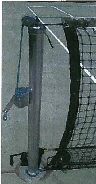
Tennis Posts and nets are to have standard 4 ½ inch diameter posts, galvanized, with a nylon rubberized net and net tightening wench mechanism to meet regulation play criteria.
