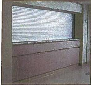
All smaller sized doors to be manually operated with a chain-hoist. If the door size is so large as to dictate the need to be motor operated, the architect needs to obtain District approval in writing.
