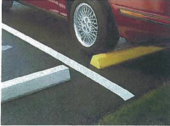
Wheel stops are to be used only in non-student parking lots. Use 4 to 6 feet long (minimum) concrete wheel stops to control traffic flow and stop cross lot traffic by vehicles. Secure to asphalt or concrete paving
