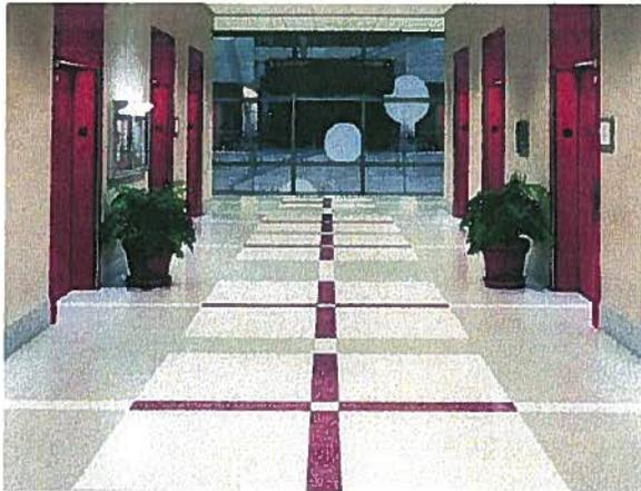
Terrazzo is a composite material poured in place or precast, which is generally used for floor and base applications. It consists of marble, quartz, granite, glass, or other suitable chips mixed with a binder that is cementitious or chemical or a combination of both. This mixture is poured on a floor with or without a base, then cured, ground and usually polished to a smooth surface. (There are some finishes of terrazzo that have a rough stone finish.)
