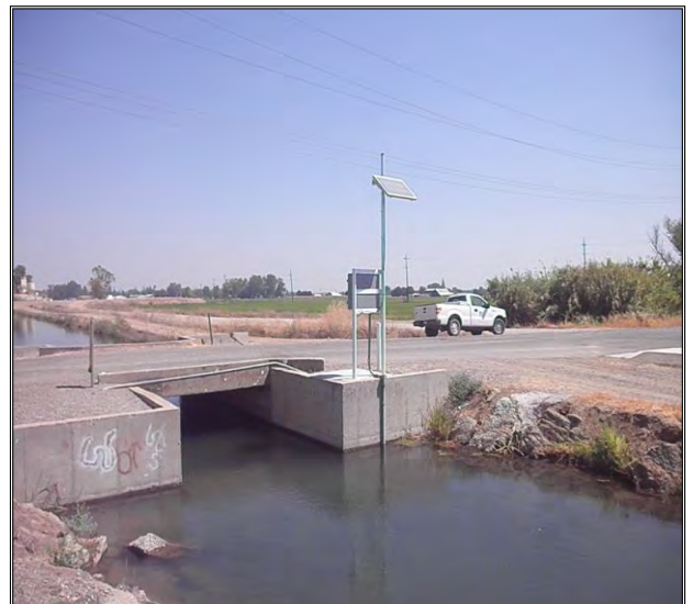
Figure 5. Looking u/s at the SonTek meter installation site along lateral 26-2 (the meter is located under the bridge)
