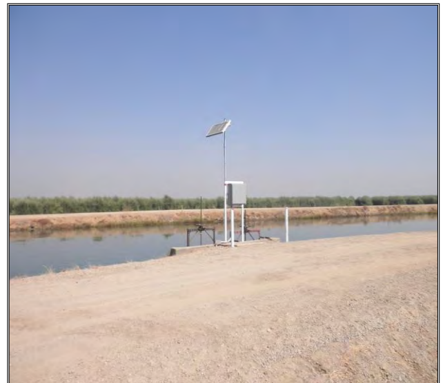
Figure 3. Looking at the head gates of lateral 21-2 off the main canal
