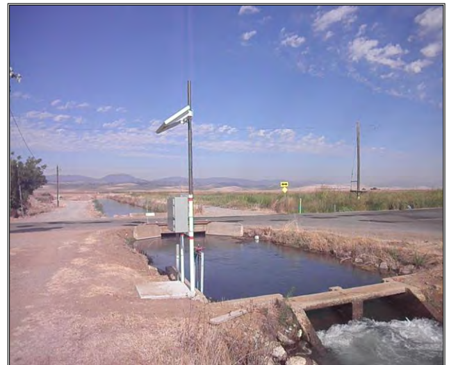
Figure 10. Looking u/s at the MACE meter installation site along Lat. 35-1 (meter is located under the bridge)
