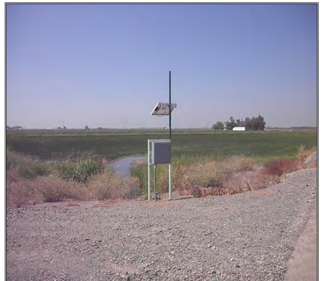
Figure 4. SonTek IQ Pipe meter location at main canal turnout 49-L
