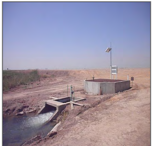
Figure 8. SonTek IQ Pipe installed immediately u/s of the control structure shown
