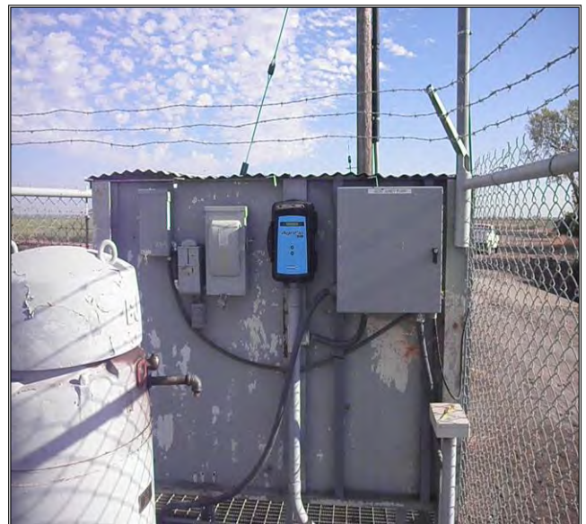
Figure 6. MACE enclosure at the Juney Weir lift pump station
