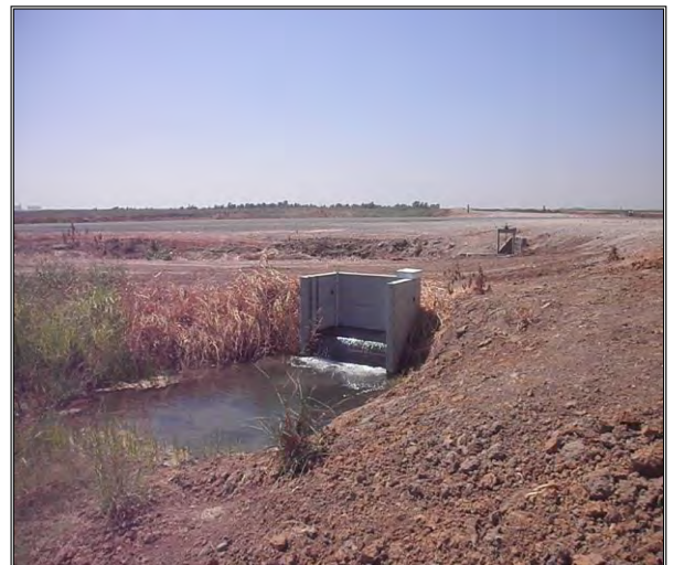
Figure 7. Lat. 28-1-1L Briggs box and sharp crested suppressed rectangular weir where the PT is located
