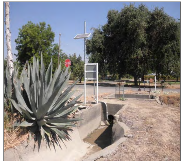
Figure 1. Looking u/s at lateral 12-3-14R
