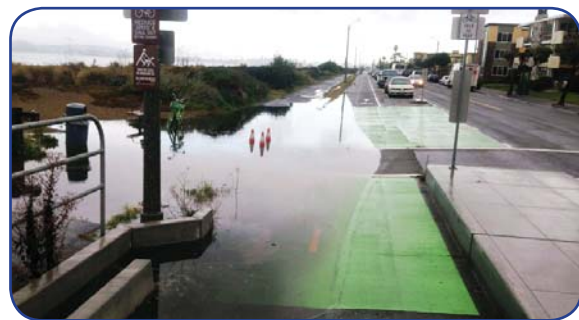
With such flat terrain and topography in our neighborhoods, the City of Alameda experiences frequent flooding of streets that also flow onto nearby properties. As shown in the City's recently adopted Climate Action and Resiliency Plan, this flooding will only grow in frequency and severity with climate change and sea level rise.
