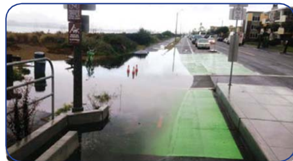
With such flat terrain and topography in our neighborhoods, the City of Alameda experiences frequent flooding of streets that also flow onto nearby properties. As shown in the City's recently adopted Climate Action and Resiliency Plan, this flooding will only grow in frequency and severity with climate change and sea level rise.
