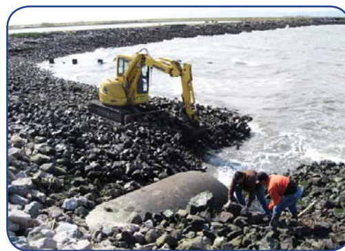
The City has conducted a series of engineering studies to determine the best ways to protect neighborhoods during big storms and sea level rise.
