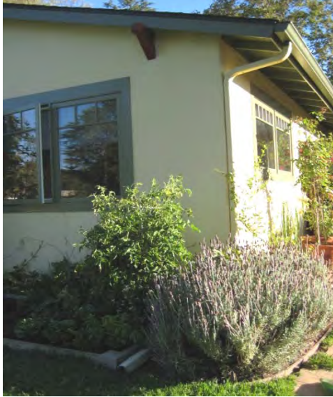
Diverted Roof Runoff City of Santa Barbara
