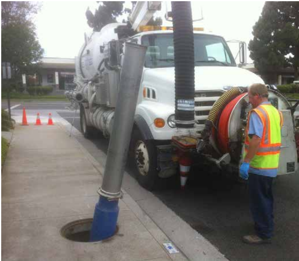
Catch Basin Cleaning Using a Vacuum Truck
