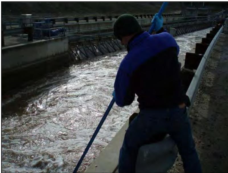
Figure 9-7. Grab Sampling Using Extended-Reach Swing Sampler
