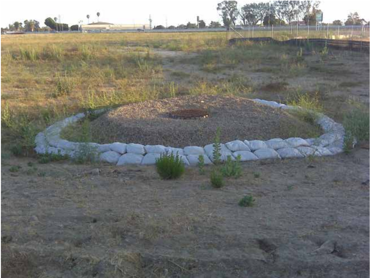
Storm drain protection during construction
