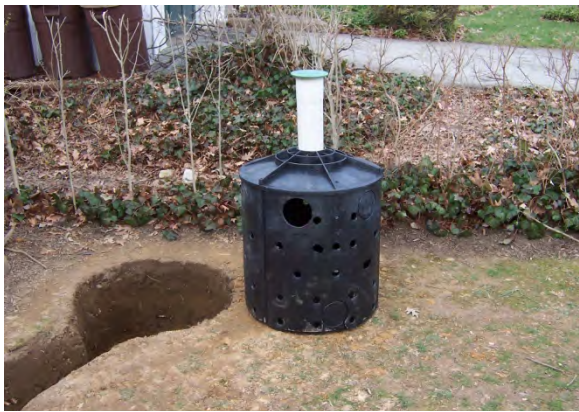
Drywell installation
