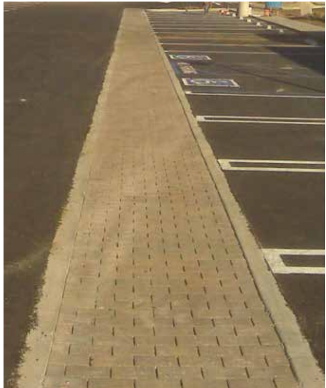
Pervious ribbon gutter in a parking lot
