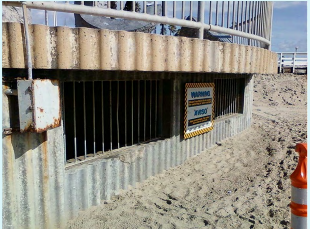
Neary Lagoon Beach Outlet Vault
