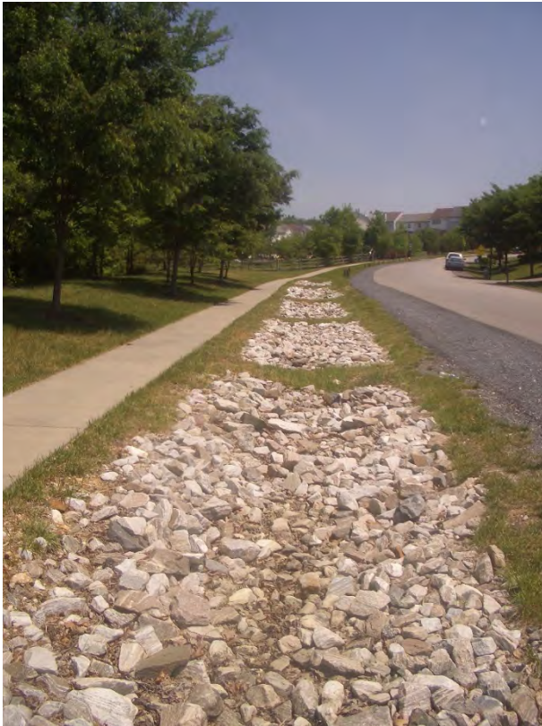
Rural Highway Infiltration Trench
