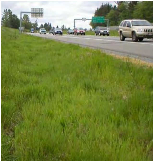
Vegetated filter strip captures runoff from freeway
