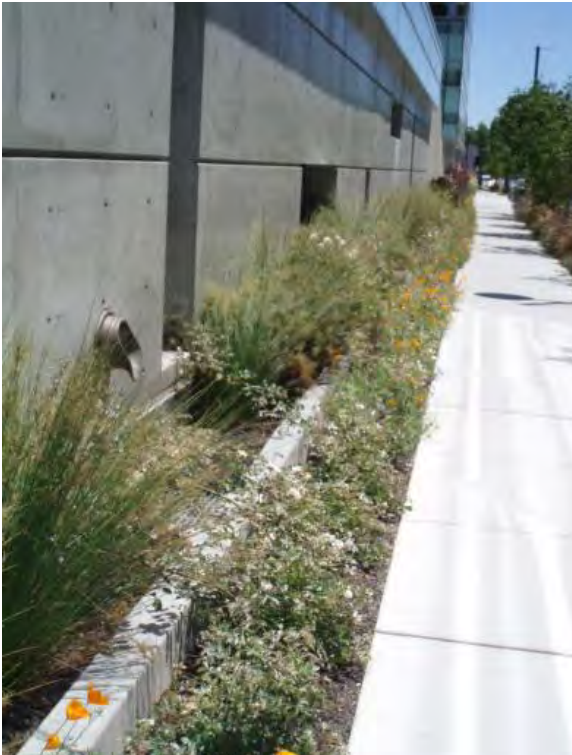
Planter boxes extending along a building wall
