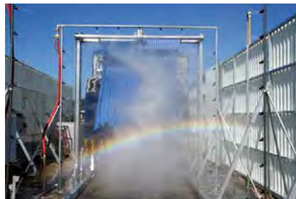
Thousand Oaks’ car wash facility that drains to wastewater treatment plant
