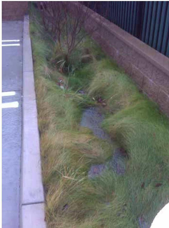
Low Impact Development infiltration BMP
