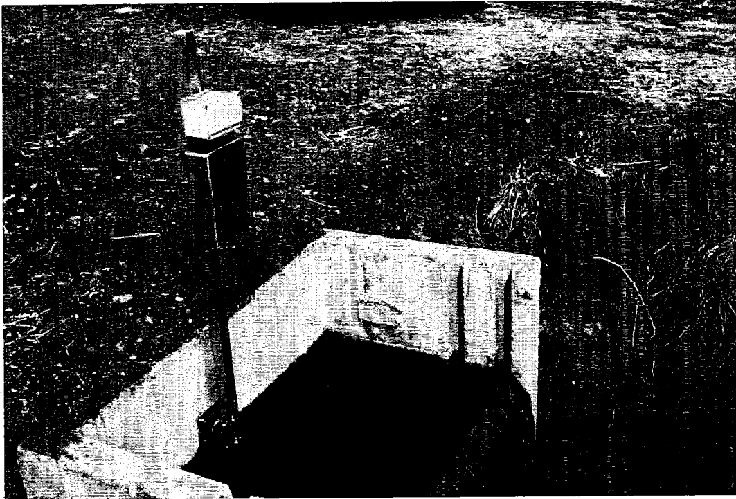
Figure 10. RemoteTracker Wireless Water Velocity Sensor Deployed in Weir Box
