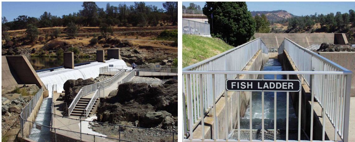
Figure 7.16 Fish Ladder at Feather River Hatchery, Oroville Dam, CA (Feather River, n.d.)
